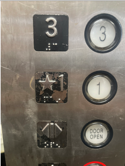
#30 Damaged Braille
